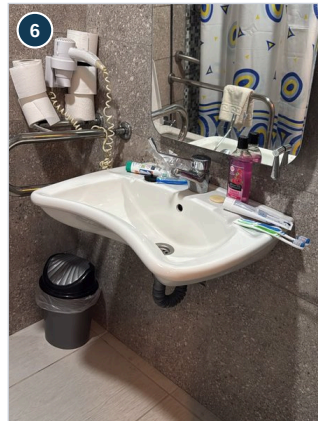
Wall-hung washbasin with open space below, lever tap and side grab bar
