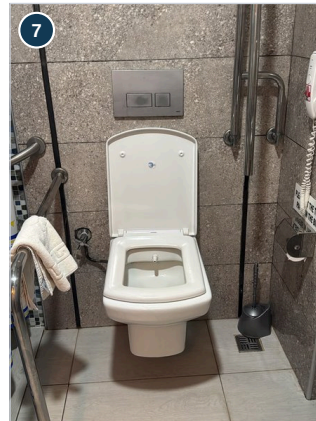
Grab bars on both sides of the toilet and wall telephone
